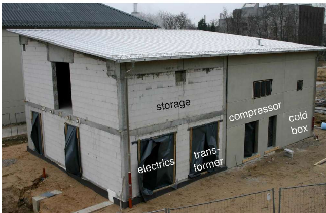
building 456 – refrigerator hall
